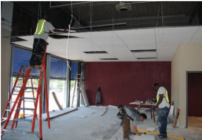
Trainees install a drop ceiling and flooring as space is prepared for the AIDS Resource Center of Wisconsin to move into a portion of the WCS Administrative Office building.
